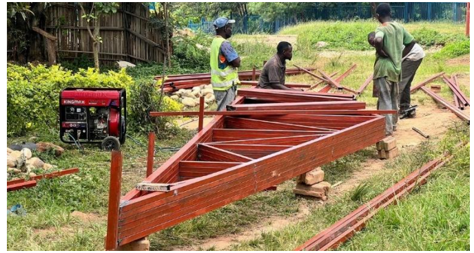
Trusses are now ready to be mounted.
